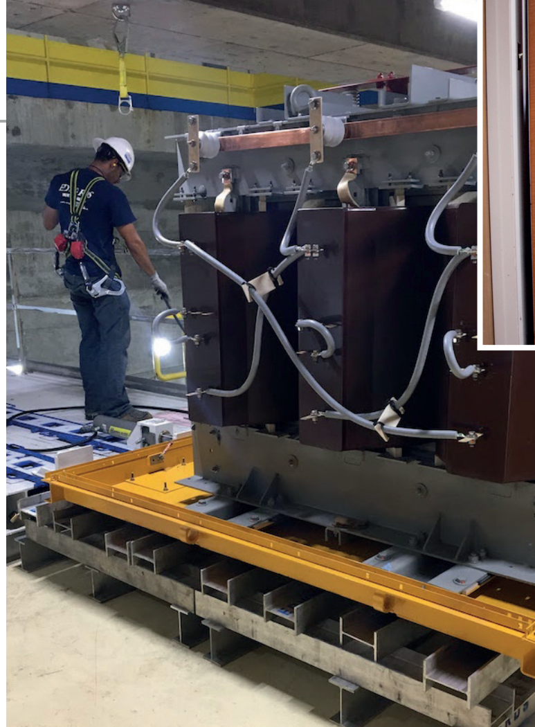
Edwards Moving & Rigging use the XLP150 with 20 ft. of track and power it with a Hydra-Pac synchronous 10,000-psi hydraulic power unit.
